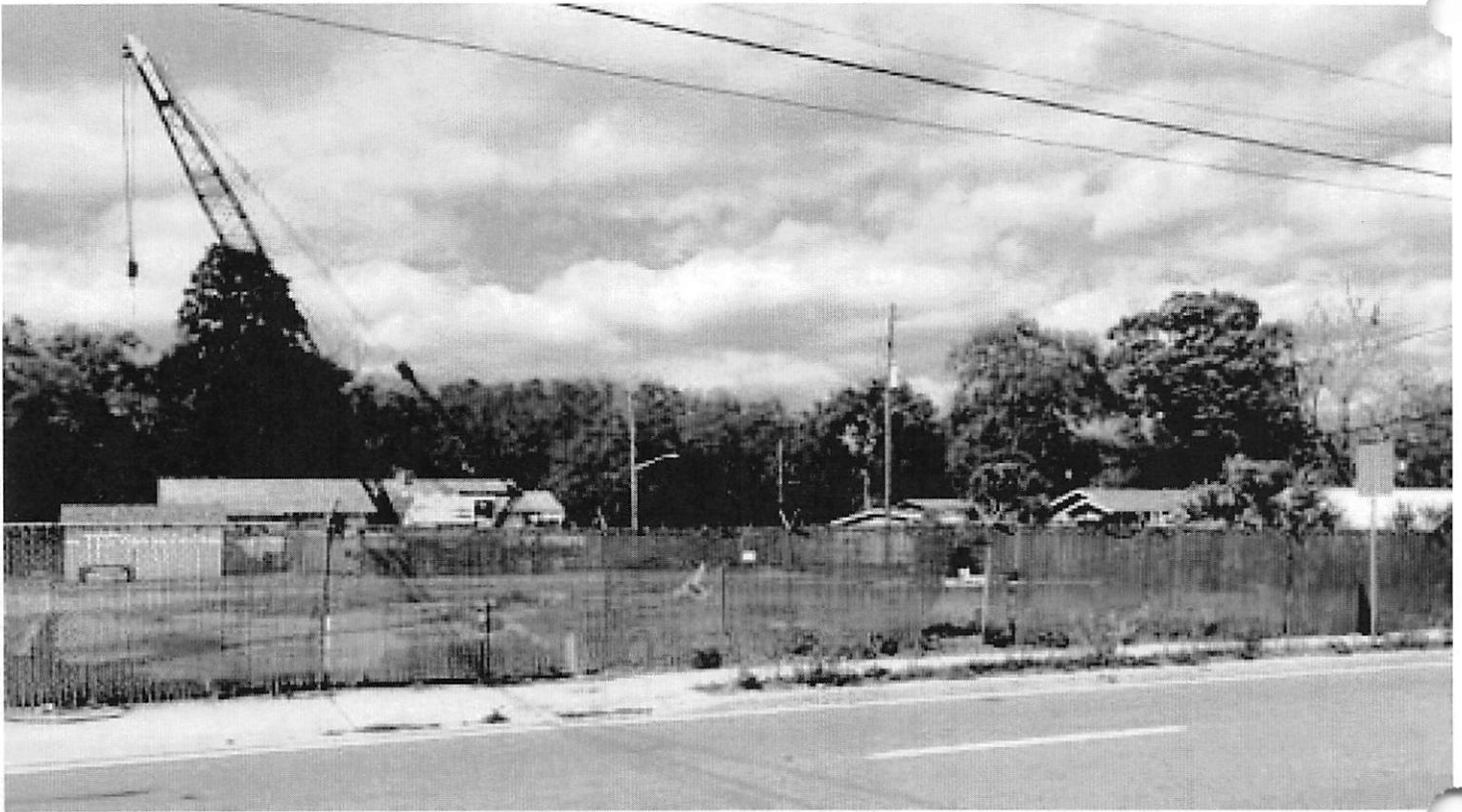
Facing northeast into the subject site from 8th Street E.
