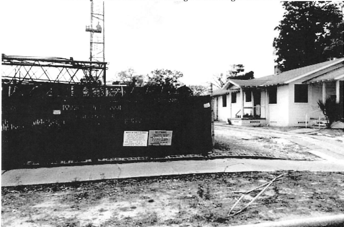
The subject site facing west from Buckman St.
